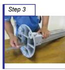
Raise the beam from the bottom of the foot approximately 30mm, to allow for height adjustment later in the assembly.
